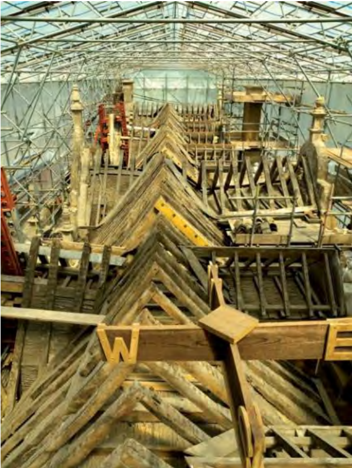
Figure 1 The east range of Apethorpe Hall, Northamptonshire, protected from the weather by a scaffold roof during English Heritage's comprehensive programme of conservation
